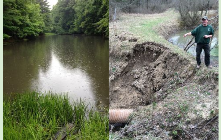
Left: Marrek Pond before dam failure. Right: Dam after failure.
